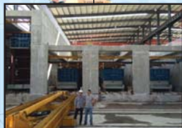
China Changchun- Mega large carrousel for precast station
